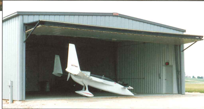
Experimental Aircraft is housed in an all-steel building with a Hi-Fold Door.
